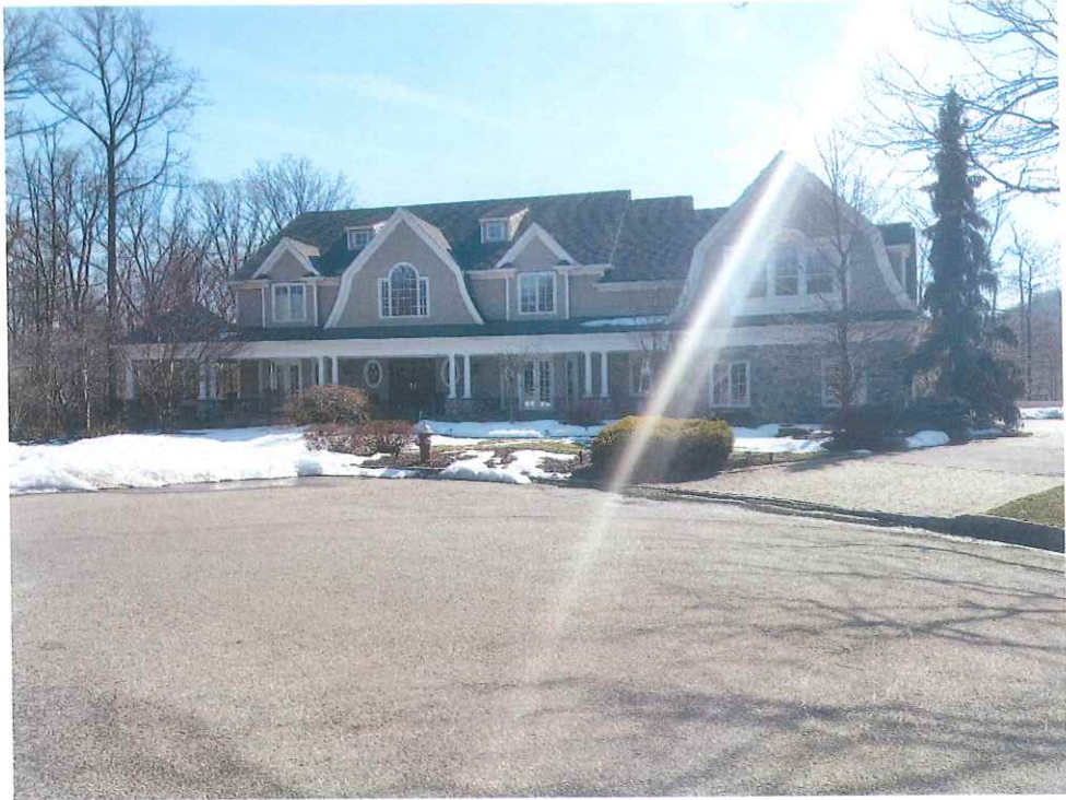
Looking south at the front of the 2-story dwelling
