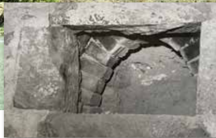
Evidence of an old Dutch "bee hive" oven can still be seen in the basement.
