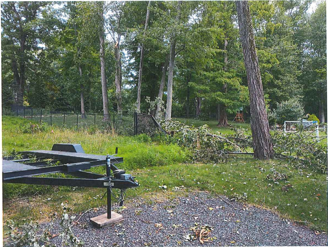
Photo #3: Looking SW from edge of driveway at storm damaged fence and rearyard
